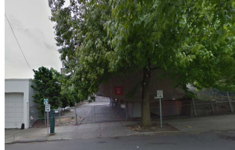
The decommissioned 157 Roy St. substation includes a barricaded driveway leading to a parking lot with space for 10+ cars.
