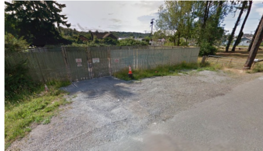
Old substation in SW Seattle with secured fencing and parking along fence-front.
