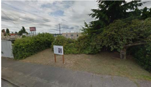
Former Aurora Substation is located adjacent to a commercial strip and a residential neighborhood.
