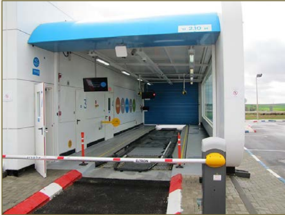
Better Place battery swapping station pilot in Israel. The exchanges were slated to cost $500,000, less than half the cost of standard fueling station. Compact in design, they could be integrated with existing fueling stations space permitted. Source: Wikimedia Commons
